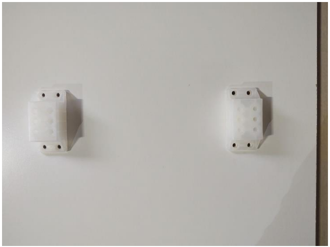
2.- Place the spacers where the holes are.
